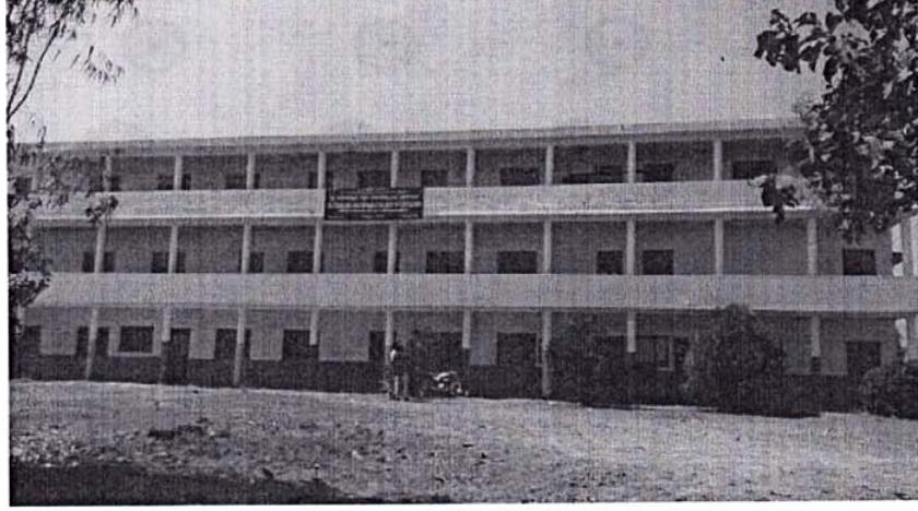
Front view of the Building
